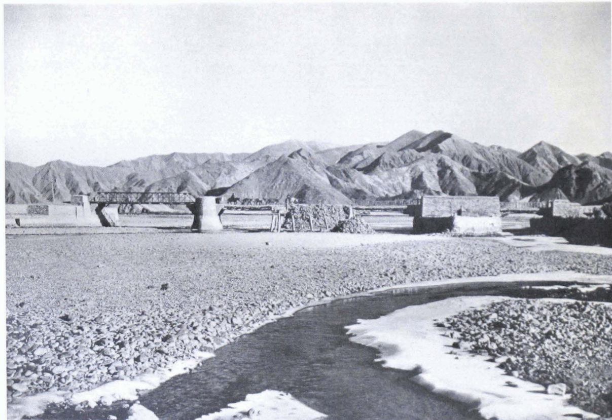
Tri-sum bridge in February. Notice modern girder arch on left and ancient cantilever arches on right
